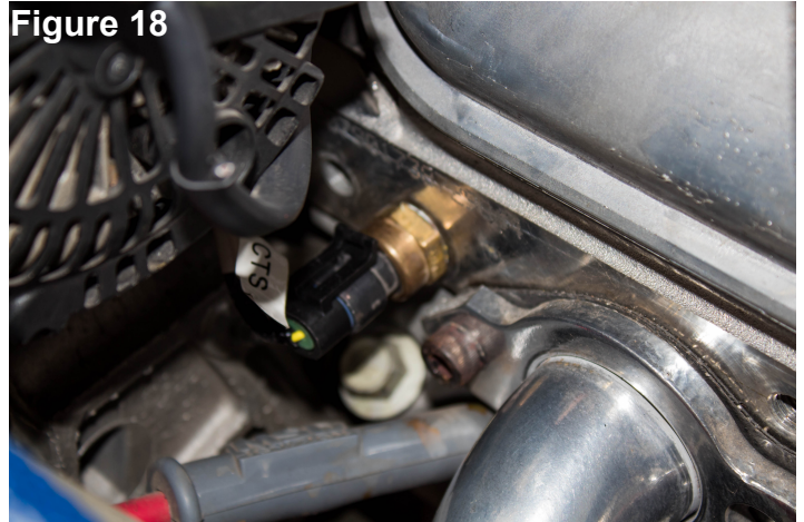
Above - The CTS connector on the main wiring harness is plugged into the Coolant Temperature Sensor in cylinder head.
